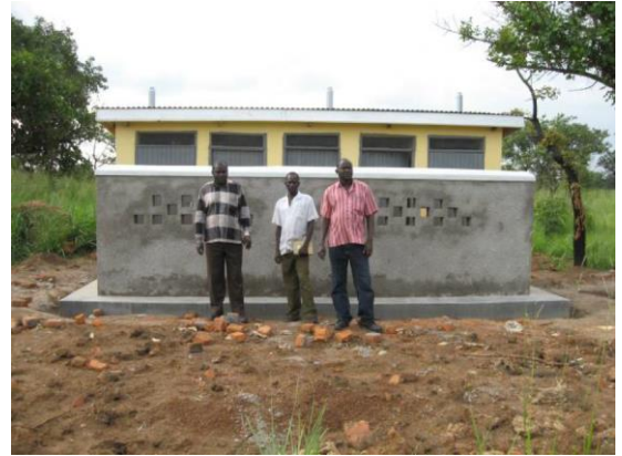
A newly constructed VIP pit latrine block at Te Gweng primary school.
